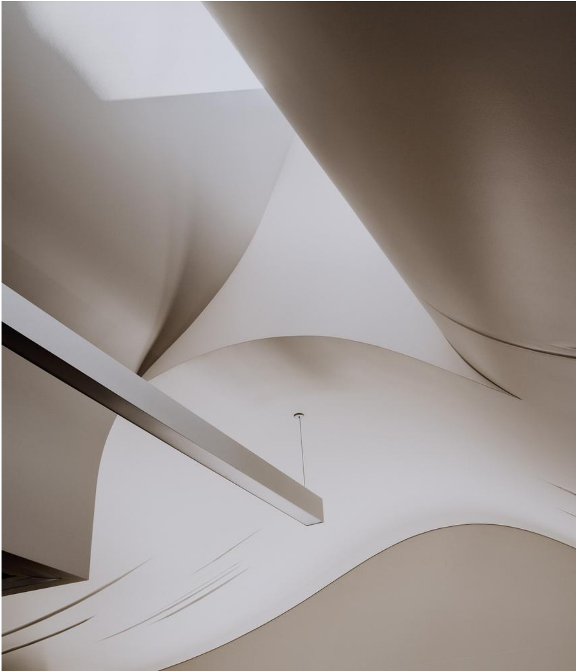
WAVE THEORY | A section of the glass-fiber-reinforced gypsum ceiling in the new kitchen. PHOTO: MARK MAHANEY FOR WSJ. MAGAZINE
